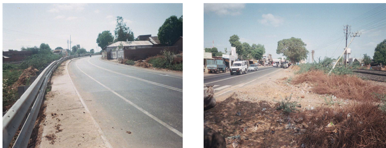
Figure E.10-3 Near Sachana Village at 47.9 Chainage
