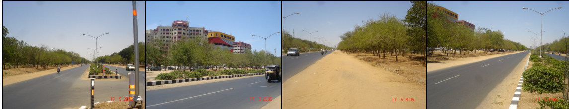
View of existing development at S T Depot near station location
