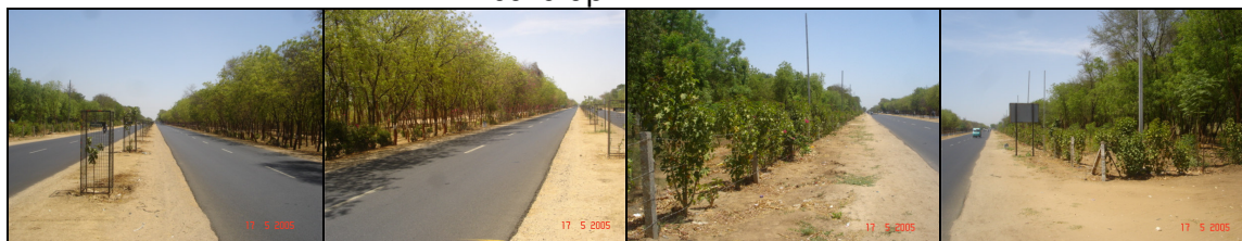
View at station Location Available space for entry/exit stairs within the greenbelt
