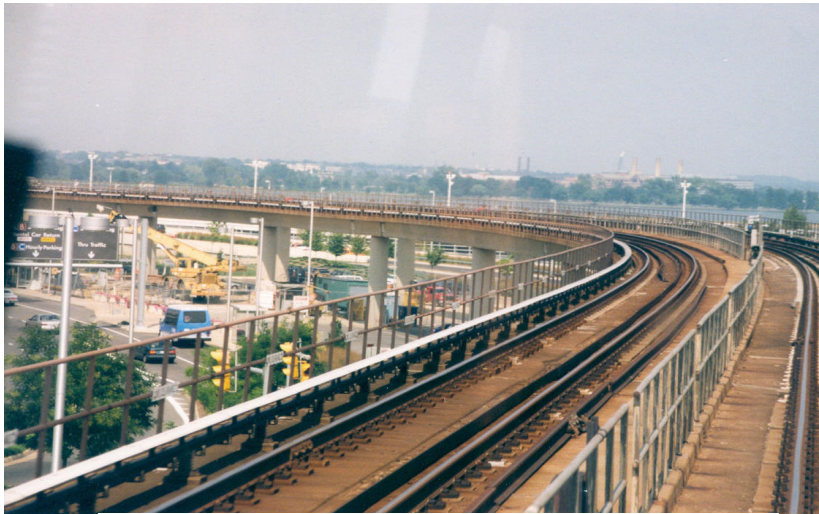
Figure 1 Picture of 750 V dc Third Rail on Elevated Viaduct
