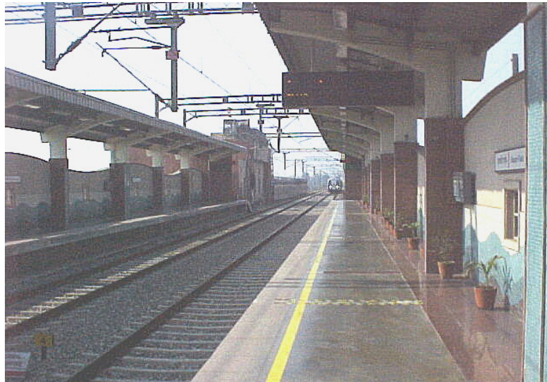
Figure 2 Picture of 25 kV ac Catenary Wires & Masts
